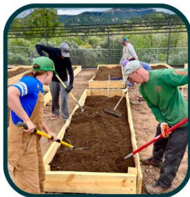
Irrigation installed and beds prepared
