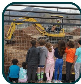
Water & electric lines installed
