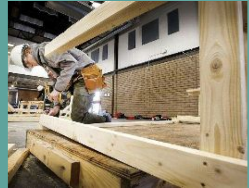
Behind the Drywall June 3-7 PCC - Mancos
